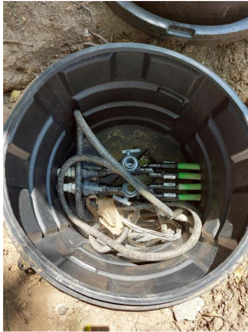
Figure 7. Manhole for connecting the BHE pipes with the underground pipes towards the container and the thermocouples' cable for temperature measurement in the borehole
