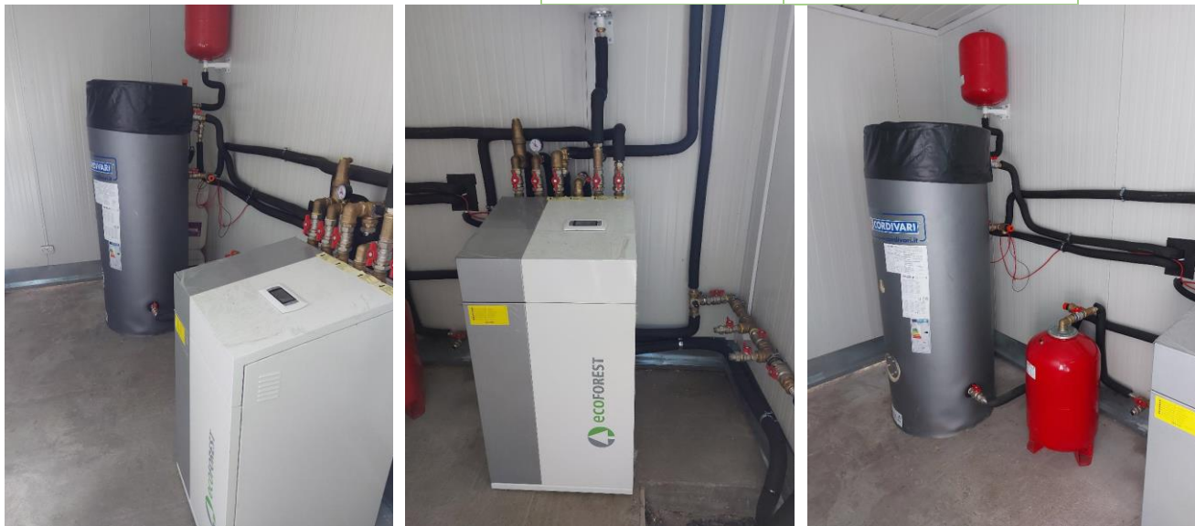
Figure 6. Final setup of the heat pump within the container
